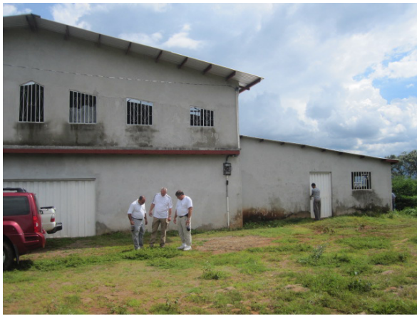
the church facility at El Renuevo
